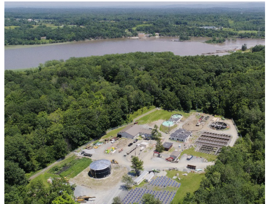
Above: The Town of Niskayuna's 3.5 million gallons per day (MGD) wastewater treatment facility.
