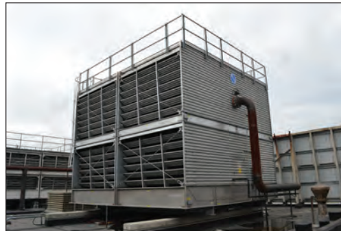
New Cooling Tower on Chiller Plant Roof
