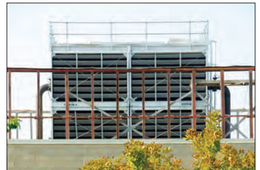
New Cooling Tower on Chiller Plant Roof
