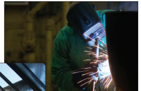
Welding Pipe for New Cooling Tower
