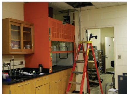
Fume Hood under construction
