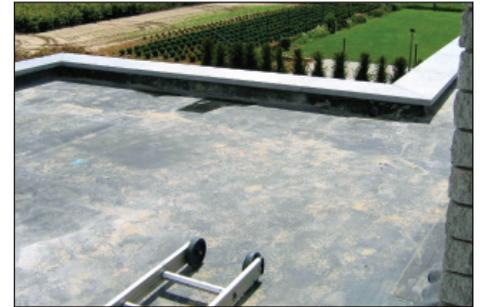
An EPDM roofing surface being installed on a flat roof.
